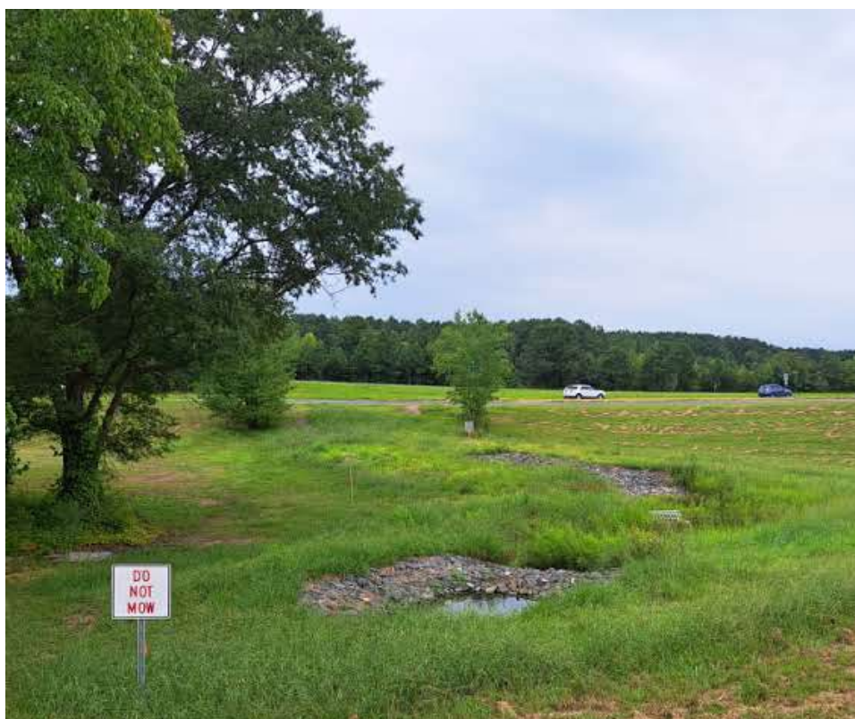
Figure 1-2. Option 2A: Constructed Wetland - Examples of Constructed Wetlands with Native, Non-Invasive Plants.
